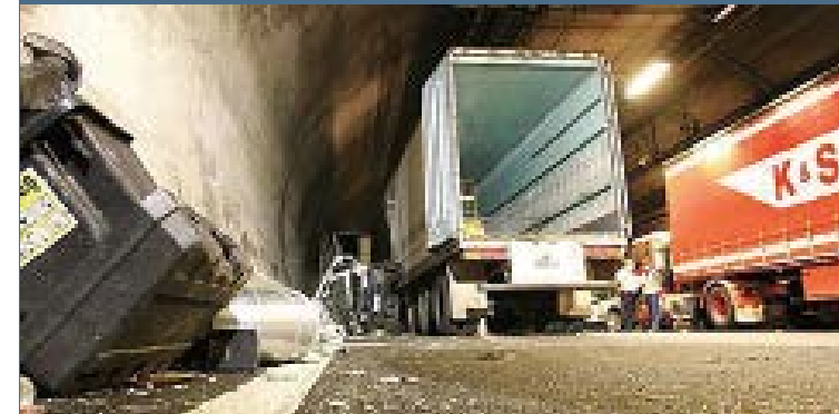
With a fixed fire fighting system installed
